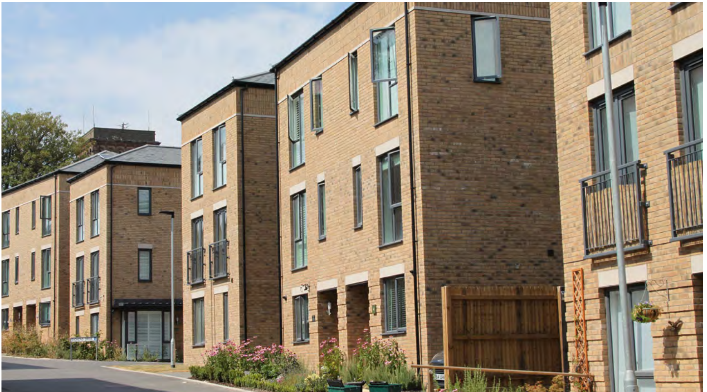
Figure 1.3d: Larger suburban developments, of up to 25 homes as covered by this guide, may result in the creation of a new suburban street with a mixture of flats and houses.
