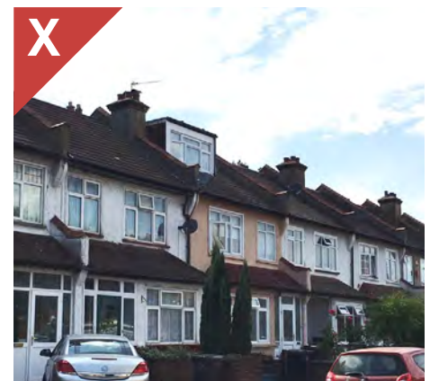
Figure 4.21f: Example of an inappropriate addition of a front dormer to a mid-terrace house. This addition lacks design merit and breaks the uniformity of the roofs that contributes to the positive characteristics of the street.
