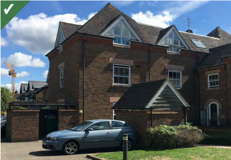
Figure 2.31b: Refuse and cycle stores that are separate from the main building but integrated into the design of the proposal through the use of the same materials and architectural features. They are situated in a discreet location with minimal impact on the streetscene, neighbouring and residents outlook.
