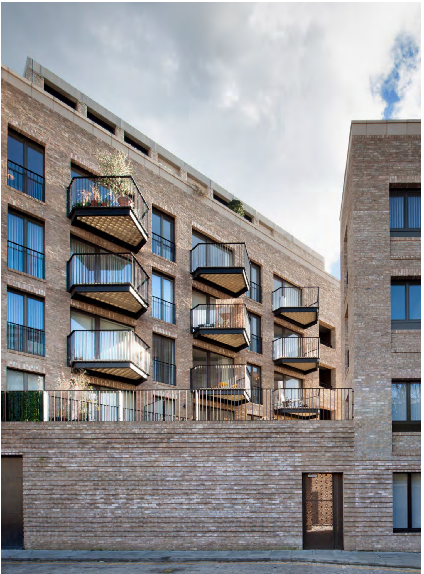
Figure 2.6f: A development of flats designed by Haworth Tompkins that uses the form of the balconies to add interest to an otherwise simple but well-designed facade giving character to a contemporary proposal. (Photo: Philip Vile)
