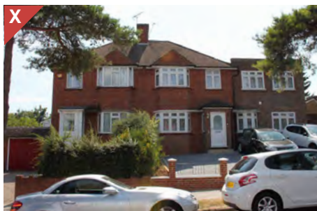
Figure 4.17b: A low quality two-storey side extension which is overly dominant, upsetting the balance of this pair of semi-detached homes. The brick neither matches nor distinguishes from the existing and the junction at the eaves is poorly detailed.
