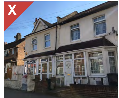
Figure 4.14b: A poor example of two porches that have been built up to and over original bay windows. The design fails to respond to the historic pattern of development and materials are low quality.
