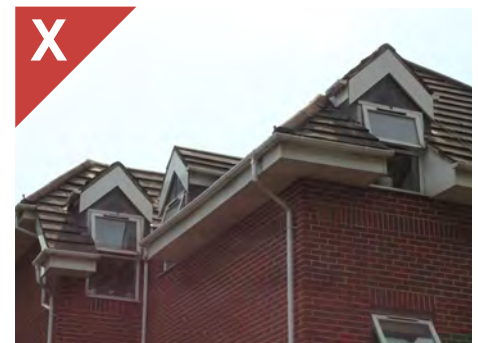
Figure 2.19h: Poorly proportioned and positioned dormers and eaves results in a poorly resolved roof.
