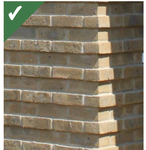
Figure 4.27e: Stepped courses of brickwork.
