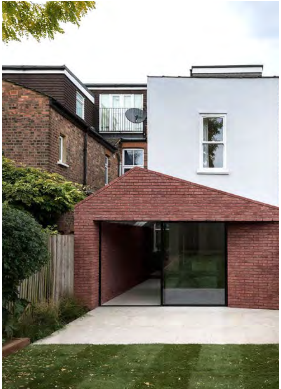
Figure 4.1b: An extension that successfully uses contemporary details and an un-symmetrical roof pitch to add interest to this design by Trehwela Williams. (Photo: Simone Bossi)
