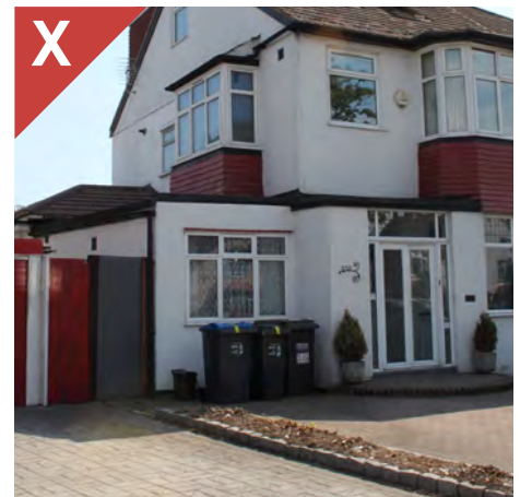
Figure 4.12b: A poorly designed single storey side extension that fails to respond to the original dwelling. It has an awkward combination of roof forms and the appearance is further exacerbated by the porch extension, which hasn't been combined with the side extension.
