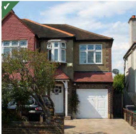
Figure 4.17a: A good example of a setback at first floor on a two-storey side extension.
