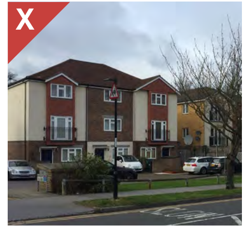
Figure 2.24a: Proportions and positioning of windows add to horizontal emphasis of the façade and contribute to a weak pastiche.
