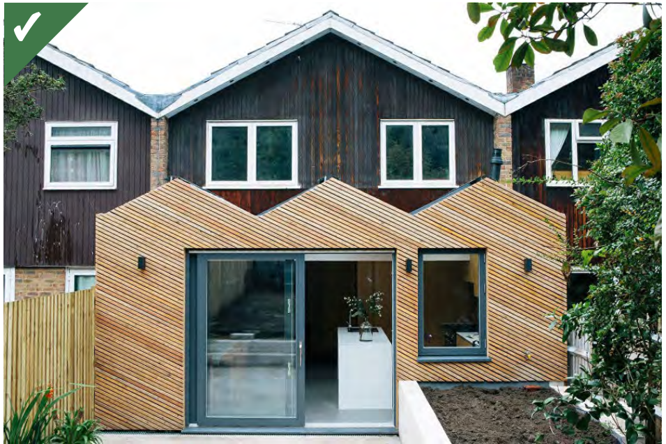
Figure 4.15a: An example of a roof design to a single storey extension by Nimtim Architects that has been designed to ensure it doesn't overlap with the windows above. (Photo: Anna + Tam)
