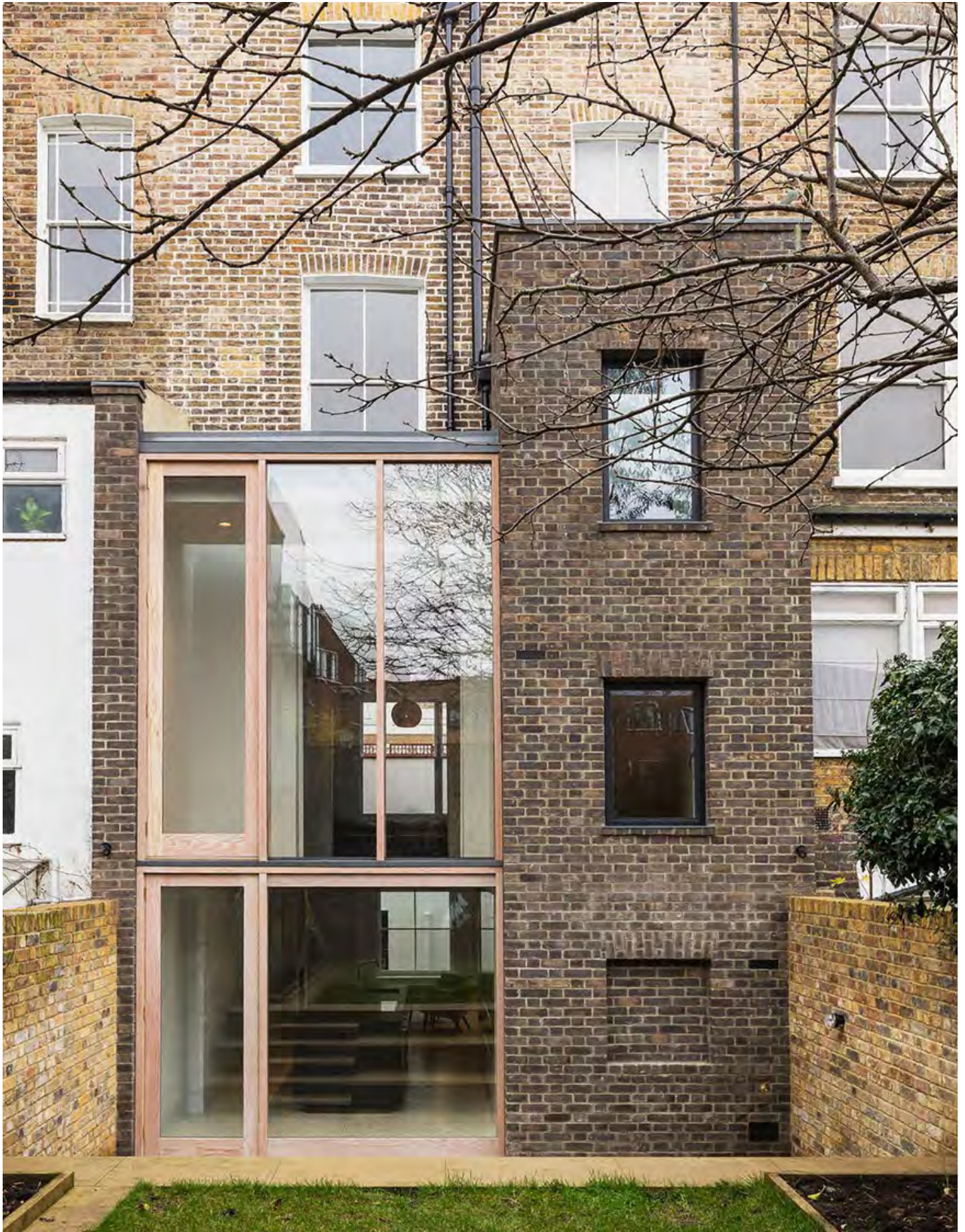
Figure 4.16a: Example of a two-storey rear extension of a terraced house designed by Gundry+Ducker Arch. that infills between existing extensions and outriggers, refer to Section 4.16 for guidance. This scheme also features a well-designed parapet detail to the roof (refer to Section 4.15) and concealed rainwater goods (refer to Section 2.24) giving a clean appearance. (Photo: Andrew Meredith)
