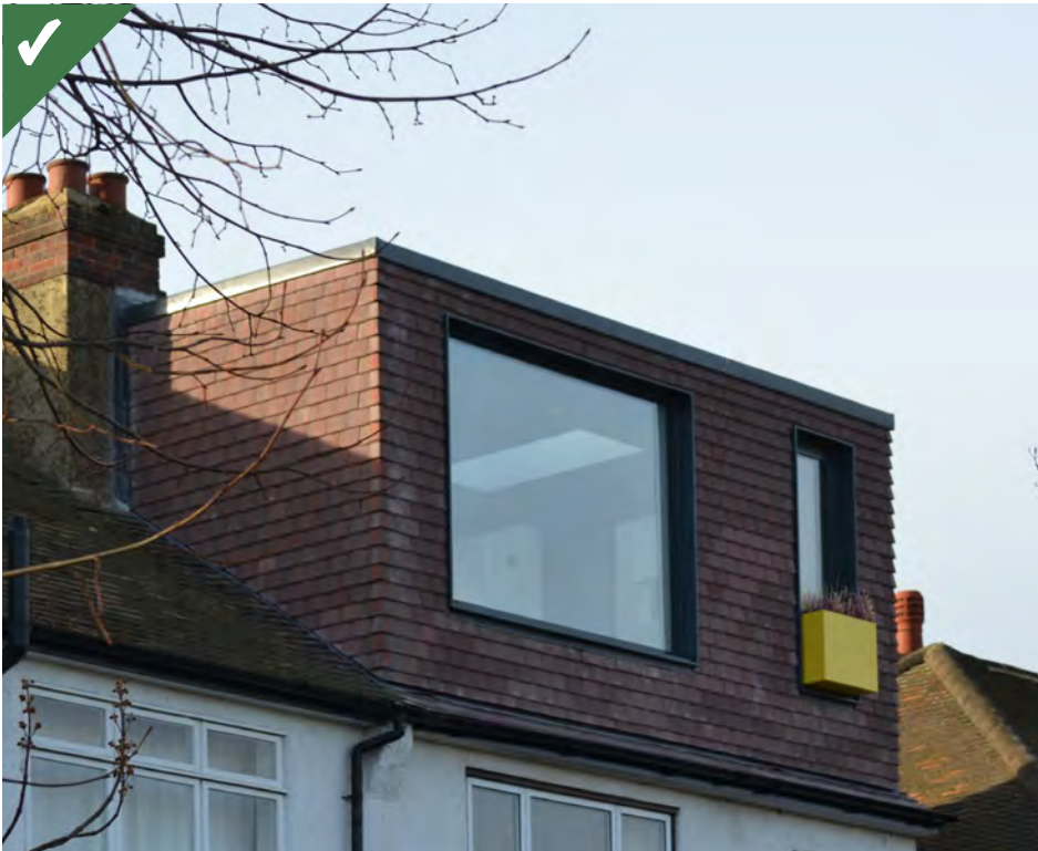
Figure 4.21c: A good example of a box dormer on the rear of a terrace house successfully designed by Selencky Parsons to integrate into the existing dwelling; the dormer replicates existing roof tiles, conceals rainwater pipes and aligns the glazing with the windows below. The dormer provides a generous amount of glazing, avoiding an overbearing appearance and benefiting the internal spaces.
