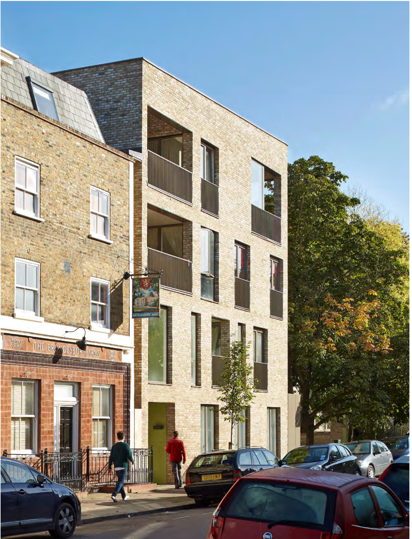
Figure 1.3e: A development of flats designed by Alison Brooks Architects within an existing residential street. (Photo: Paul Riddle)
