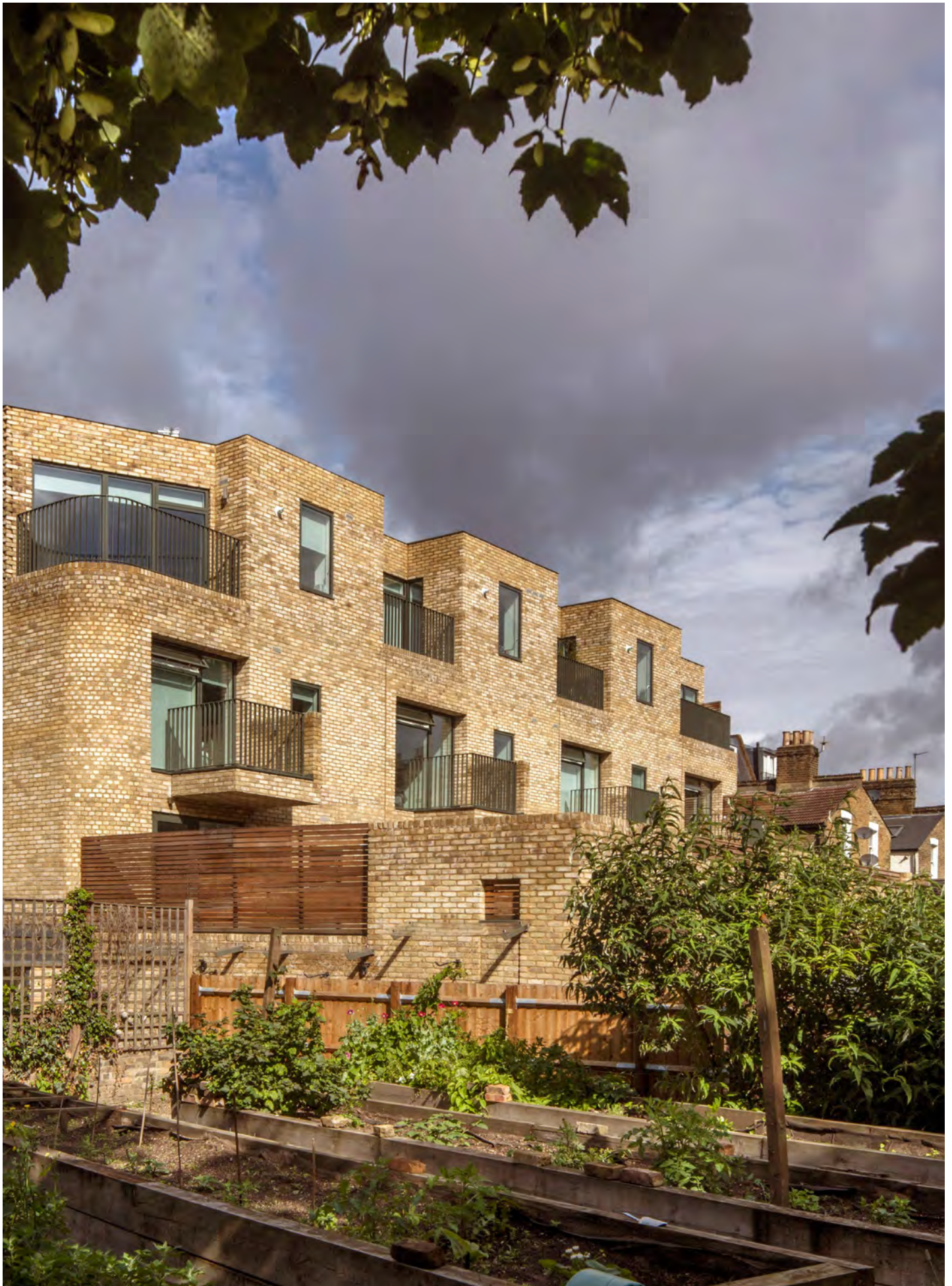
Figure 2.6e: Development of a larger scale designed by Peter Barber Architects is successfully integrated into the context through a stepped form on the top floor and careful choice of high-quality materials that respond to local character. (Photo: Morley von Sternberg)
