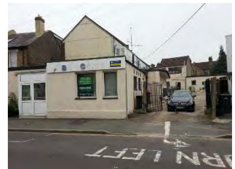
Figure 2.5a: Oval Mews, before redevelopment with a change of use.
