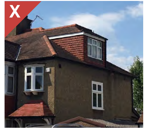
Figure 4.21e: Example of where a side roof extension to a house has not been setback from the original roof. In this situation it has compromised the symmetrical form of the original semi-detached houses and therefore negatively impacts the appearance of street.
