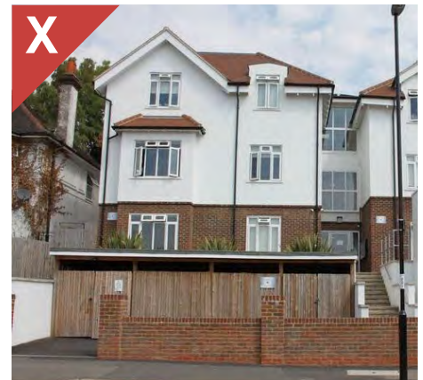
Figure 2.29b: Failure to screen hardstanding and bin stores with a landscaped boundary treatment.
