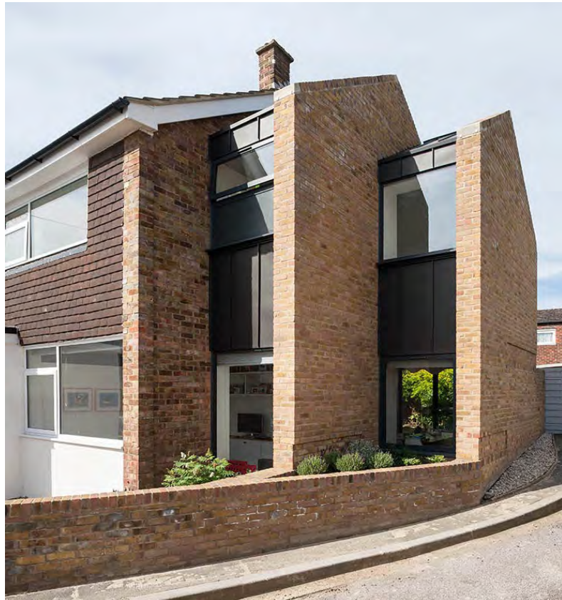
Figure 4.5a: A supplementary side extension designed by Selencky Parsons. The form clearly relates to the existing house, but successfully introduces larger windows and combines new materials with brickwork to complement the existing house. (Photo: Andy Matthews)
