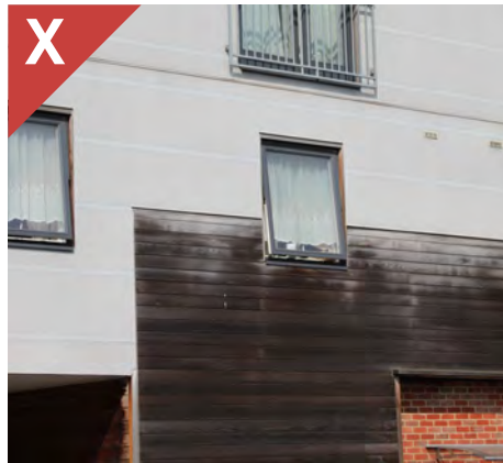
Figure 2.23i: Use of wood that weathers unevenly near material joins and has not been properly maintained.
