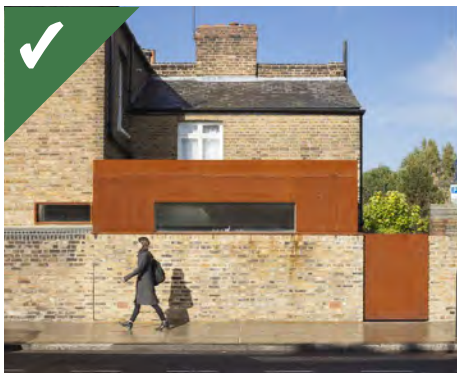
Figure 4.26c: An example of the successful introduction of contemporary materials in this metal clad side extension by HUT Architecture.
